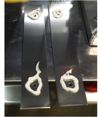
Apply silicone around each of the 4 holes
