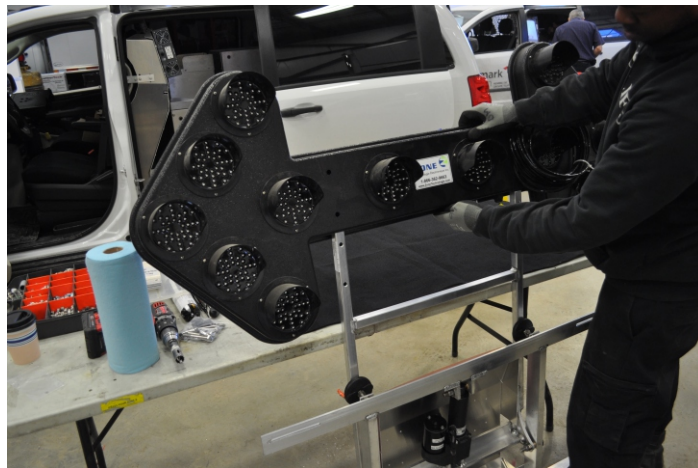
Insert the bracket into the 2 holes
